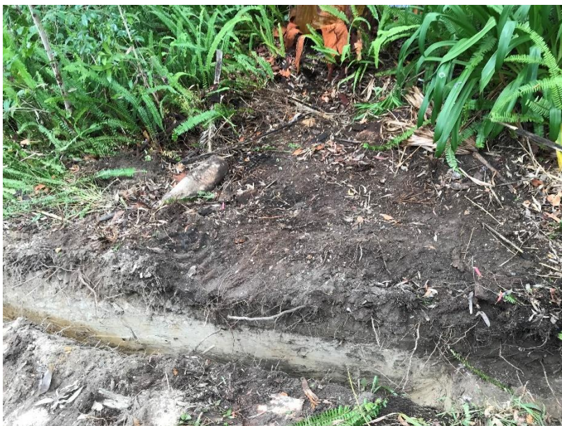
Figure 18 Face of trench beside tree 26, no roots encountered.
