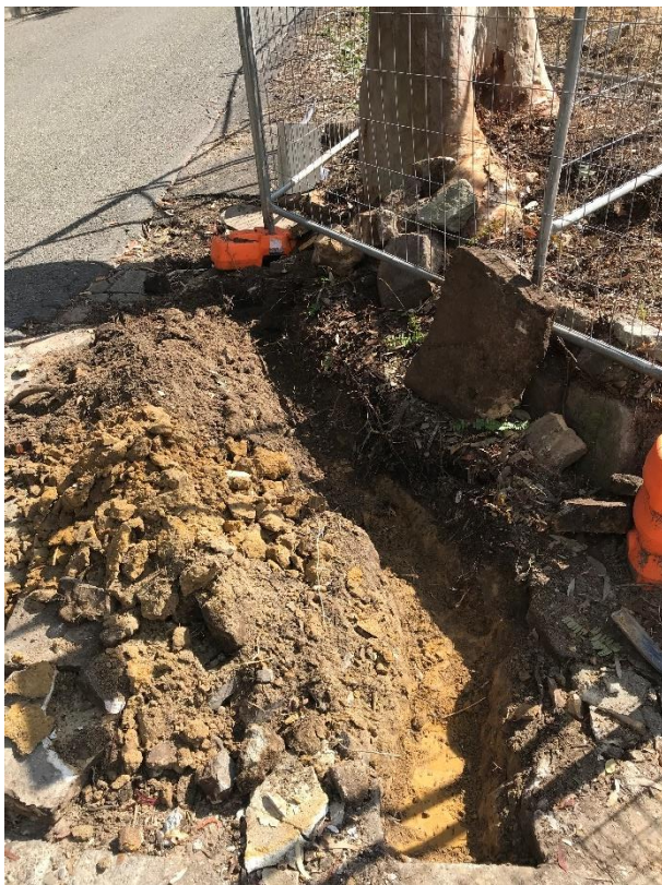
Figure 9 Lower trench 200mm deep no tree roots from tree 21
