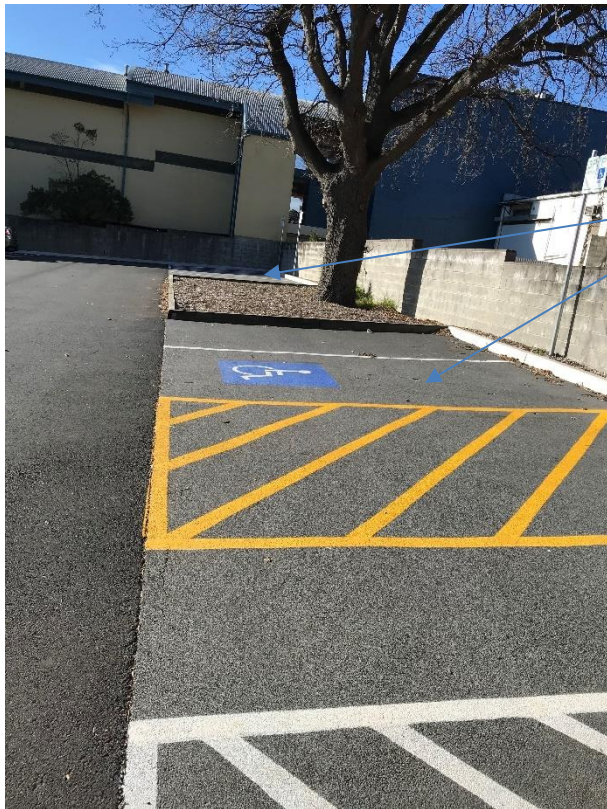
Figure 11 Stone Set and no fines concrete used to create a carpark within the TPZ of a mature English Oak at 3 Patanga Road Frenchs Forest.
