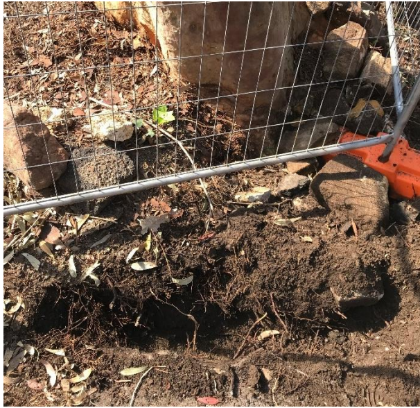
Figure 8 Up hill western trench 200mm deep, no tree roots from tree 21
