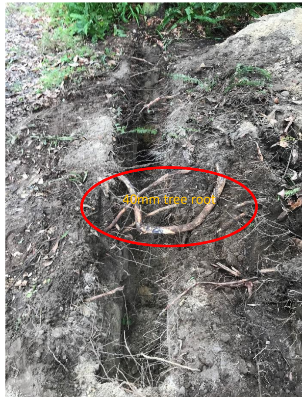
Figure 2 40mm tree root located within trench
