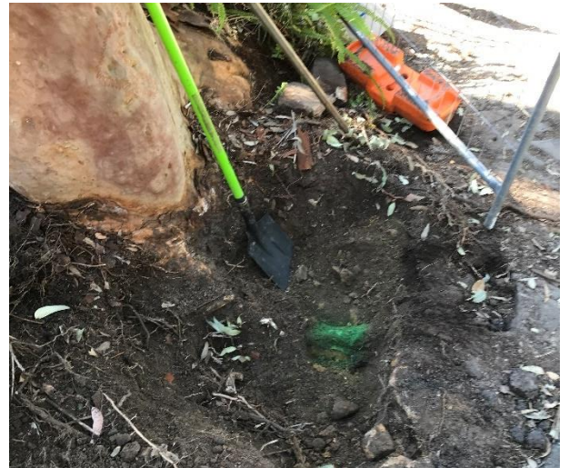
Figure 7 Middle trench, excavation between the road and tree 21. One 40mm tree root located 200mm below ground level
