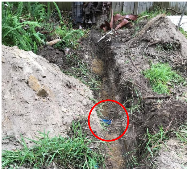
Figure 12 Tree root 110mm found 4 metres from tree 21
