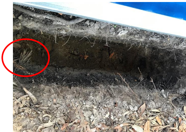
Figure 21 Northern section, 20mm tree root located.
